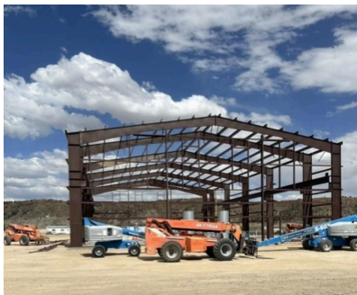
Durango Machining Innovations' new construction in Farmington.
