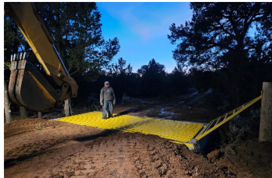
The New Mexico Off Highway Vehicle Association (NMOHVA) and the Carson National Forest El Rito Ranger District collaborated on replacing fence gates with cattle guards to support motorized use that also allows grazing permittees to keep cattle in designated pastures.
