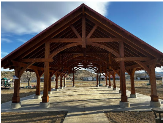
The Village of Cimarron installed a group shelter in their town park to encourage community
